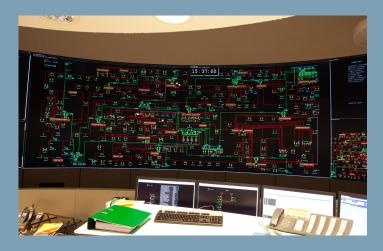
designing and deploying digital video displays in the European control room environment. With input and support by ELSIS TS, Litgrid deployed 36 Clarity LED3 Series displays (c67RP-LED3) in a twelve-wide by threehigh (12 x 3) configuration. With each display measuring approximately 53 inches by 40 inches, the total video wall encompasses nearly 550 square feet. On the ELSIS TS side, the effort was led by Ramunas Bazevicius, head of sales for the company.
